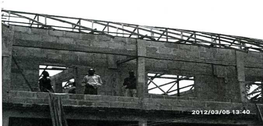
The auditorium at the roofing stage before I left home
